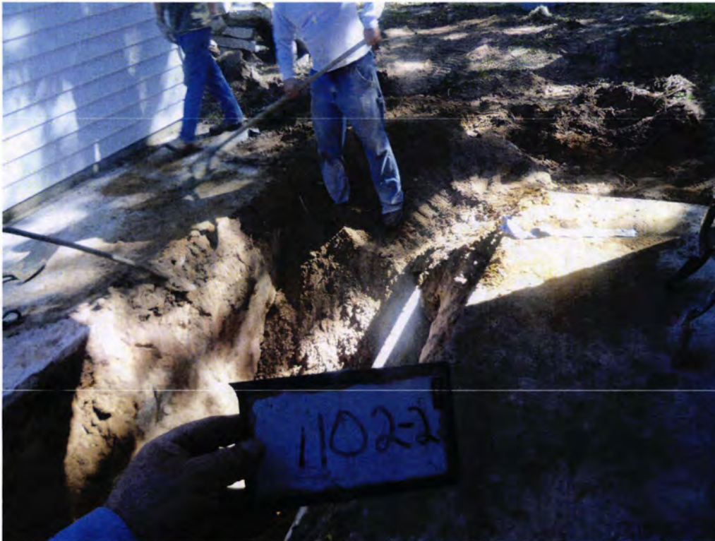
Picture 3 Excavation for UST 1102Iris-2.
