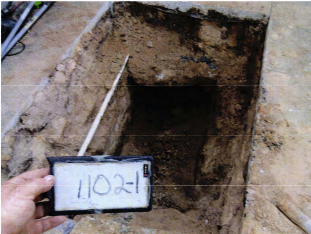
Picture 2 Excavation for UST 1102Iris-1.
